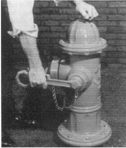
1. Remove Nozzle Cap.
