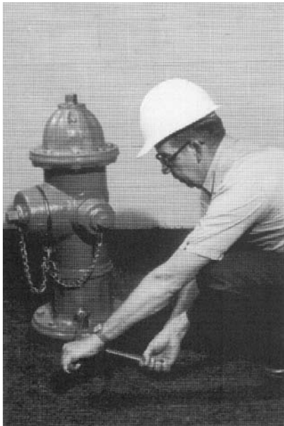
1. Loosen Nuts on Safety Flange Bolts.
