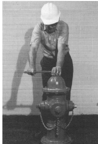
4. Tighten Operating Nut, turning in closing direction.
