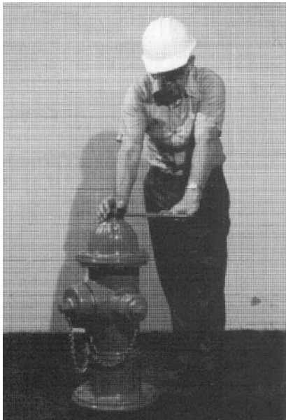
2. Turn Operating Nut slightly in the opening direction to relieve compression between Barrel sections.
