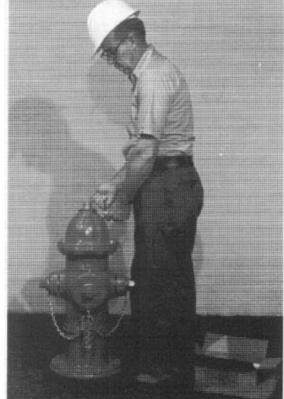
3. When oil is level with Oil Filler Plug Hole, replace Oil Filler Plug.
