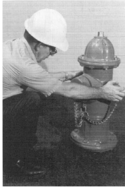
3. Rotate Upper Barrel section as desired.
